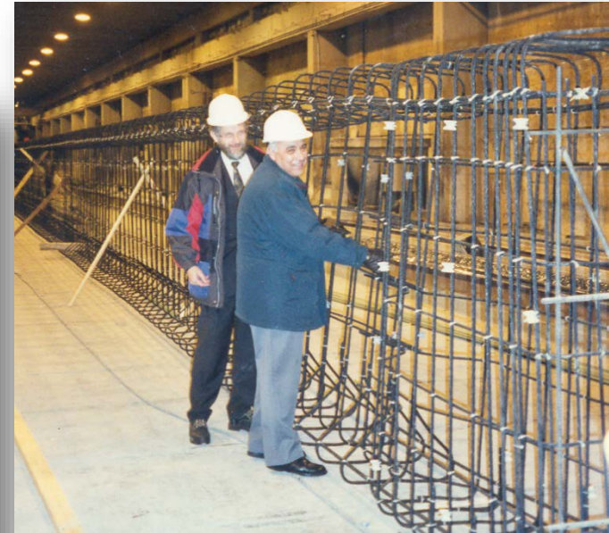
Placing CFRP stirrups for Taylor bridge girder (1996)
